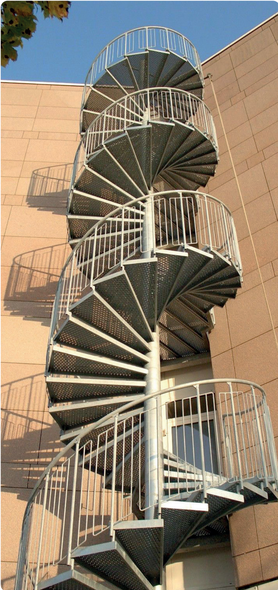
There are various surface embossings to choose from. Here: Graepel-Universal with perforated leading edge
