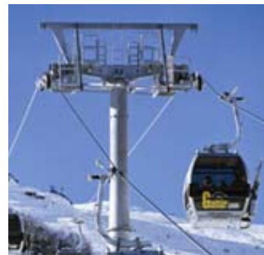
Service platforms for cableways
